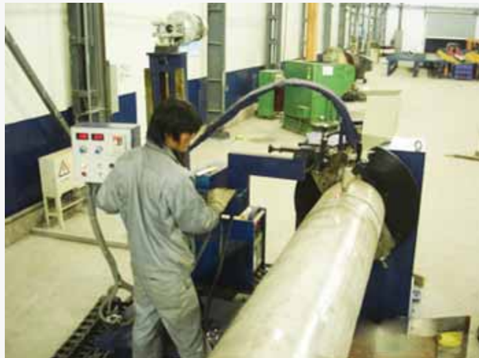
Piping Cantilever Automatic Welding Machine(SAW)
